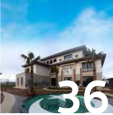
VİLLA CEPHESİNDE İSTANBUL SİLÜETİ Istanbul silhouette on the villa facade
